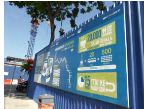
Pic 4 New railway construction
